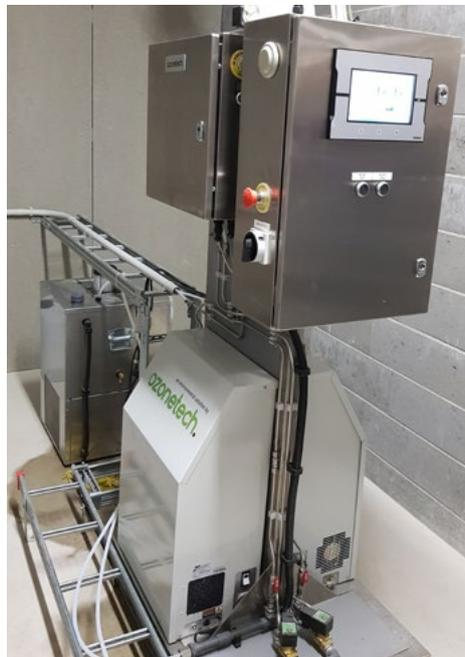
The RENA Pro C6 system with integrated cooling system installed at Tallinn Zoo.
